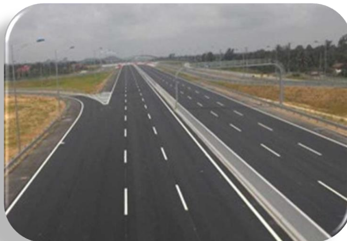
NR13 Road Improvement and Maintenance Project Lao PDR USD0.995 Million
